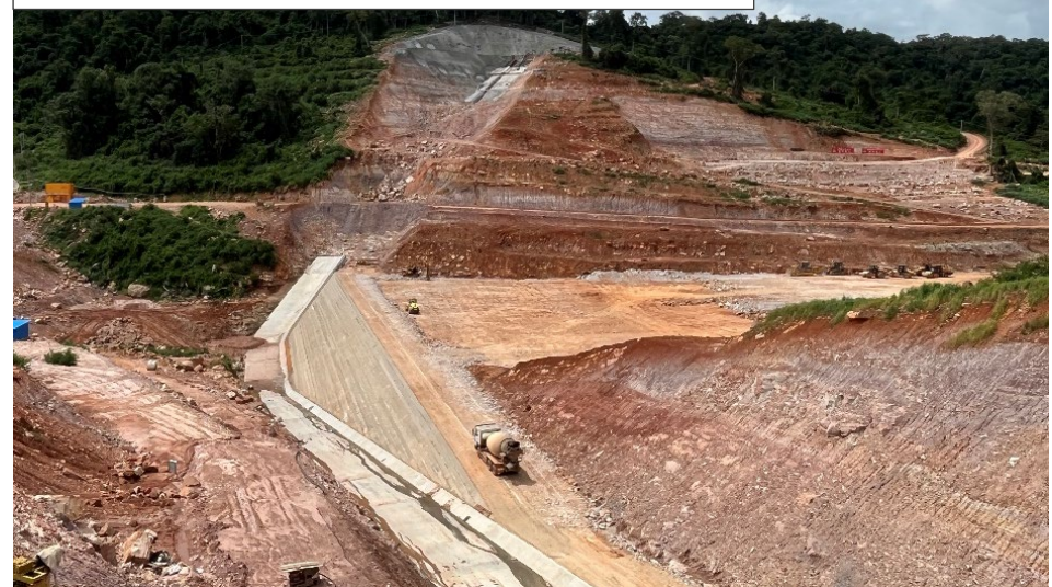
Main Dam Area (photo taken from the south)
