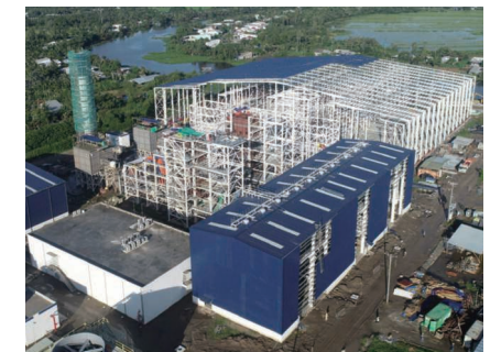
Hau Giang Biomass Power Plant under construction
