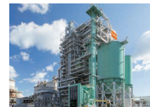
erex's first new-build biomass power plant
